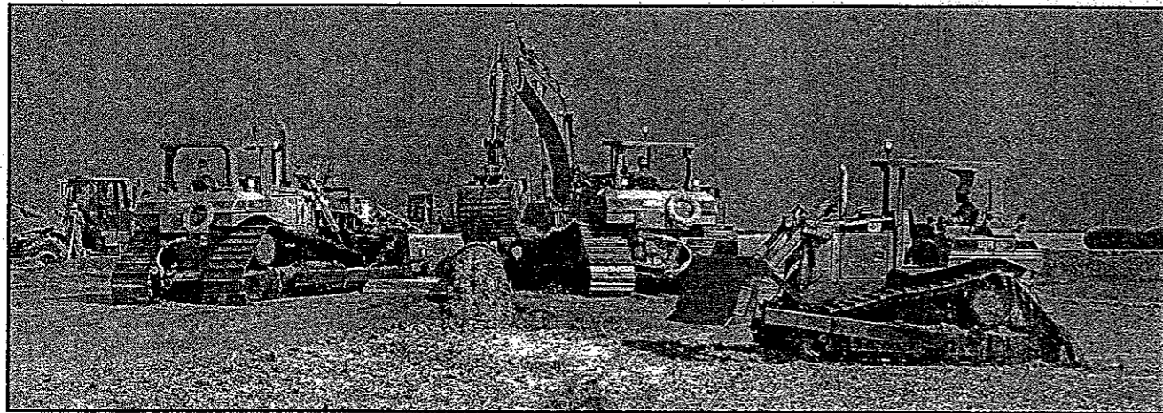
Shovels spread the sand discharged onto the platform by jumbo dredgers connected to a pipeline system. Right: Square-wheeled compactors level the reclaimed land.
